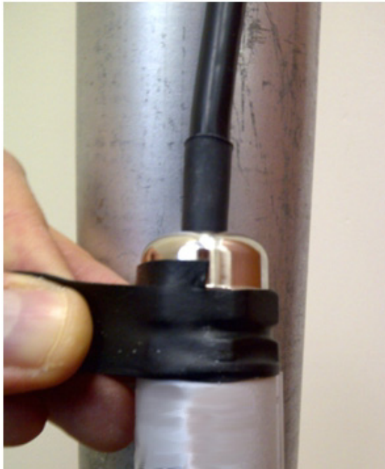
Figure 3-21: Protecting the unit joints with vinyl tape
